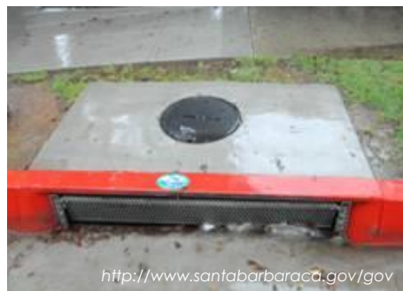
Catch basin opening screen cover
