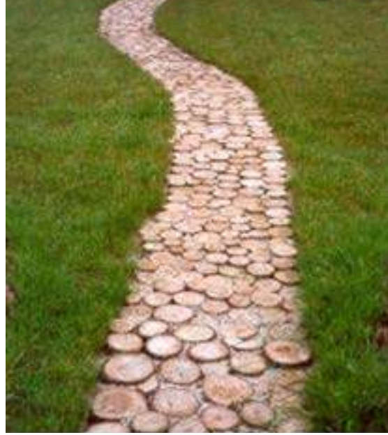
Figure 48. Cross sectional cut of palm tree trunk and pathway constructed using cuts. (Kate, 2015)
