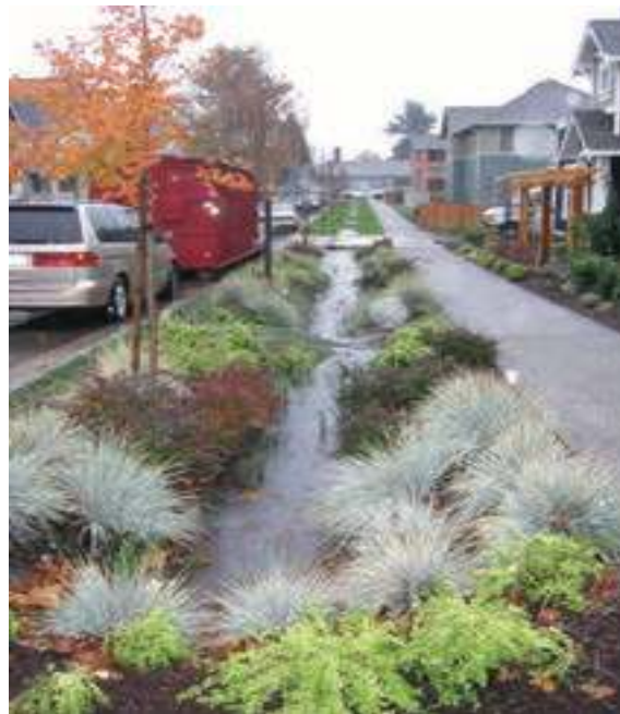
Figure 33. Bio-swale example in upstate New York. (City of Binghamton, 2021)
